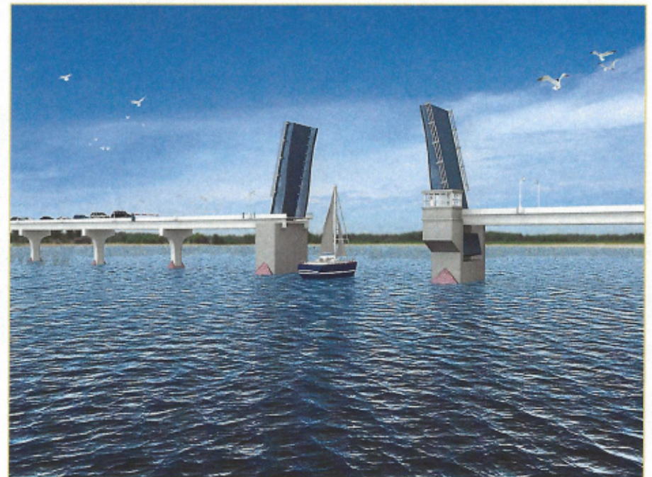
Bridge in open position
